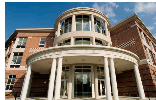
Moore Humanities and Research Administration Building
