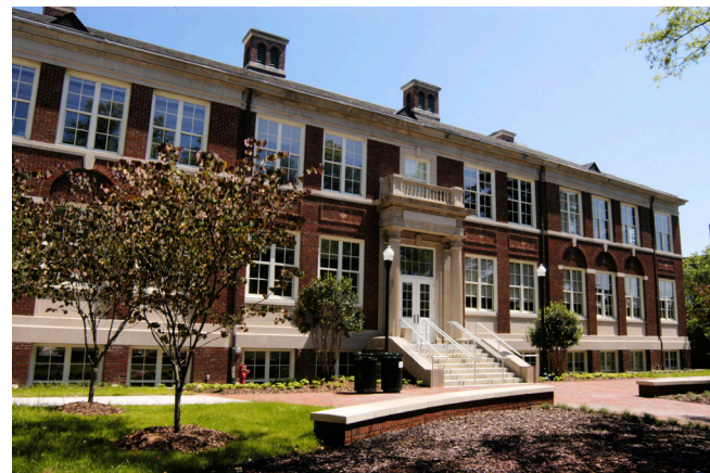
Stone Building: Appropriate use of color and materials palette
