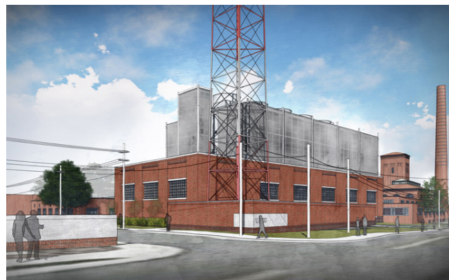
South Chiller Plant (Under Construction)
