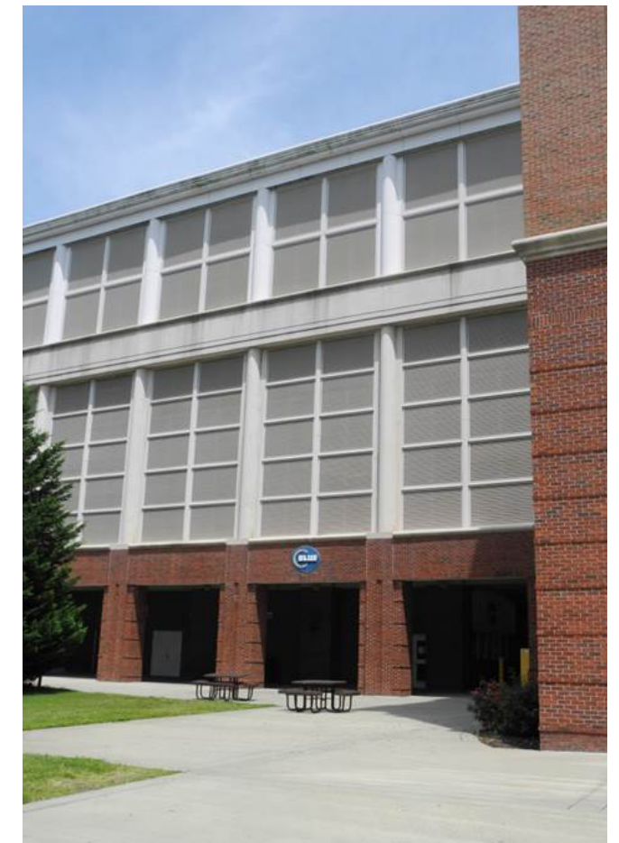
Mclver Parking Deck and Chilled Water Plant
