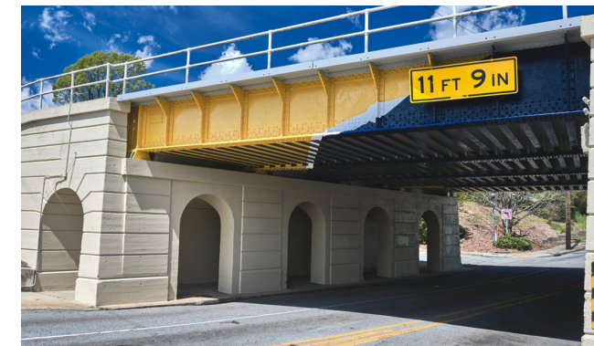
Josephine Boyd Underpass
