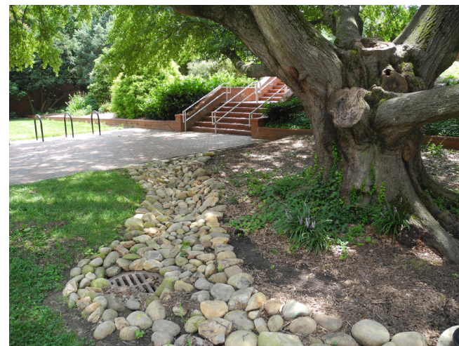
Stone culvert for stormwater management
